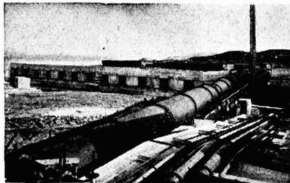
Large-bore pipes such as this sea-water main, storage vessels and ducting throughout the plant are rubber lined, and rubber again covers the huge fan units and 4 miles of steel girders.
