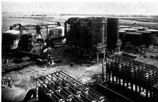
*On the left of our picture can be seen the oxidation units, comprising catalytic converters and heat exchangers; centre, SO<sub>3</sub> coolers. The acid coolers are in the foreground*
