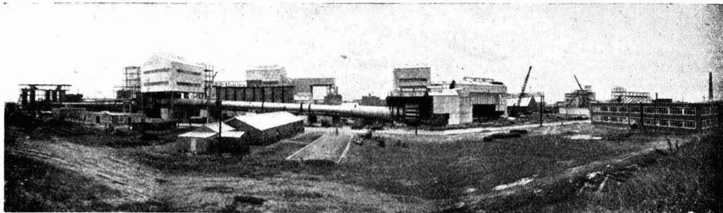
*General view of USAC's factory showing (left to right) drying and absorber towers, kiln feed house, rotary kilns, kiln firing house, clinker bunkers and the administration building*
