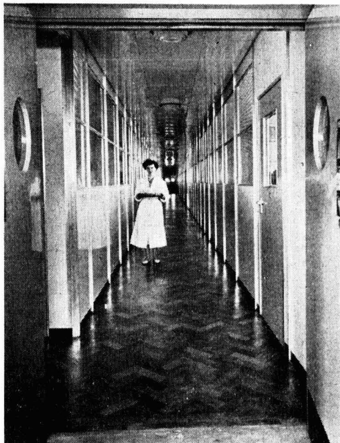
View along first floor corridor showing Frenger ceiling with recessed lighting fittings
