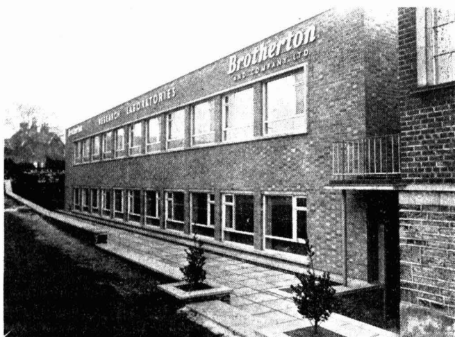
The new wing at the central research laboratories of Brotherton & Co. Ltd., Leeds
