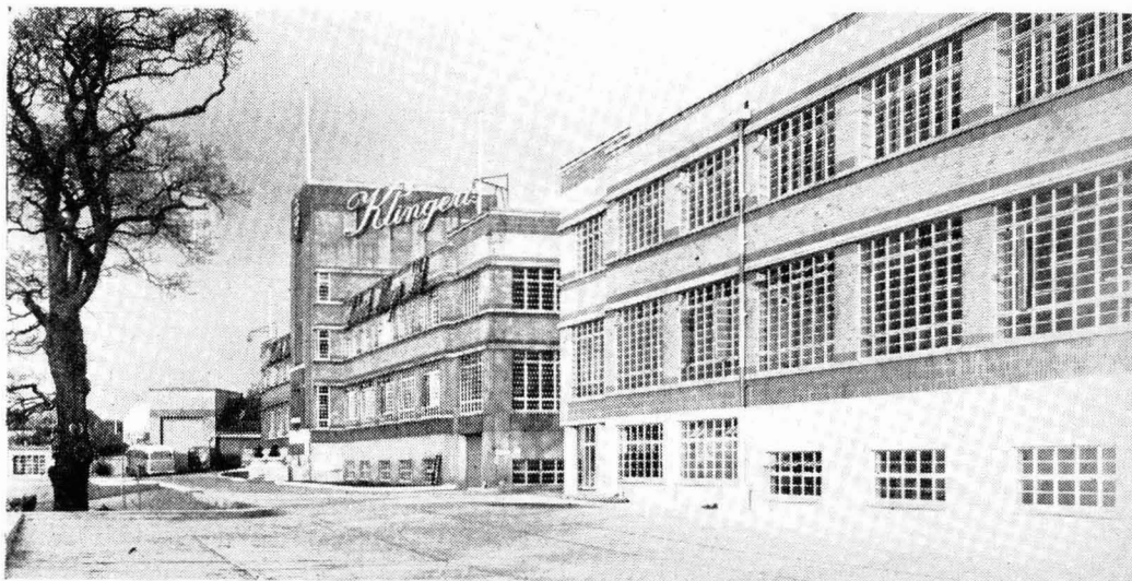
Klingerit works at Sidcup. The new wing is on the right
