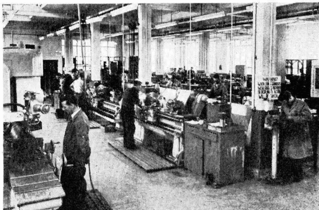
Section of the machine shop in the new wing at Klingerit works
