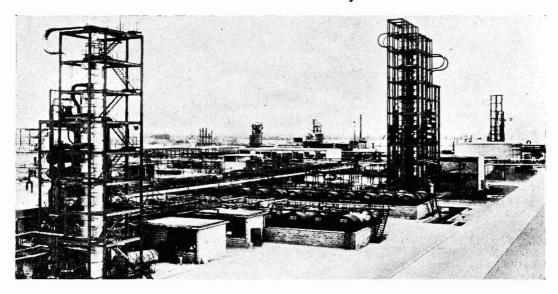
ABOVE: General view of part of the Petrochemicals plant at Urmston, Manchester, showing (left) primary distillation unit, and (right) the re-run and azeotropic distillation unit
