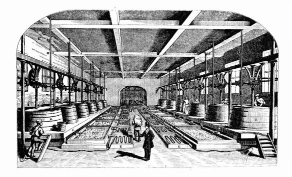
RIGHT: A row of ballingfurnaces at the Felling Chemical Works, near Newcastle (as they existed in 1844) for the conversion of sulphate of soda into ballsoda. At one stage of the process, a low four-wheeled iron carriage, bearing a shallow tray, was wheeled to the front of the furnace. The workmen then drew off the semi-fluid mass into the tray by means of a rake. Shortly after the mass had been removed, innumerable little jets of flame burst out at its surface
