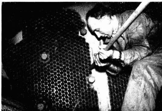
Installing titanium condenser tubes at Uskmouth Power Station
