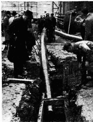
Fig. 1: Laying a nine in. diameter Alkathene drain pipe
