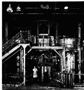
View of the plant showing the loading bay. Graphitising furnace is on the left and carbonising furnace on the right
