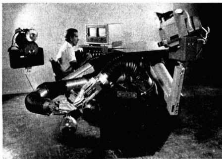
Light touch of the Mobot Mark II is illustrated by this photo, in which the machine prepares to pour liquid chemical from one flask to another
