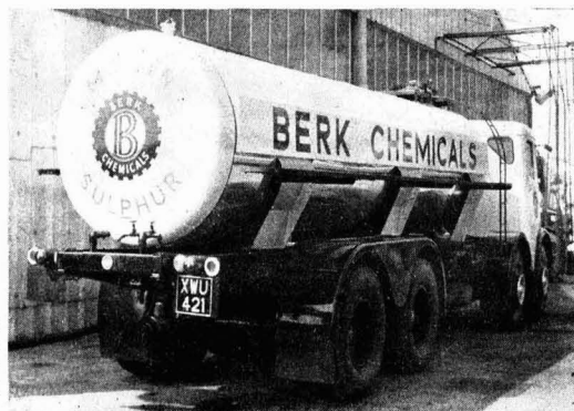
One of the Berk fleet of road tankers for the transport of molten sulphur
