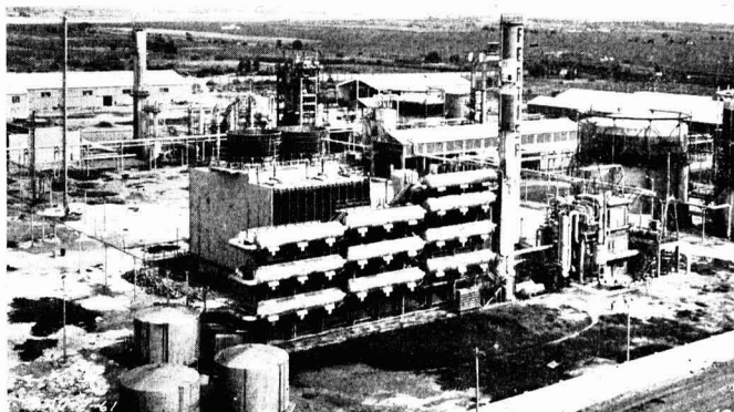
The plants of Fertilizantes Sintetico S.A. built at Callao, Peru, by engineers of Montecatini
