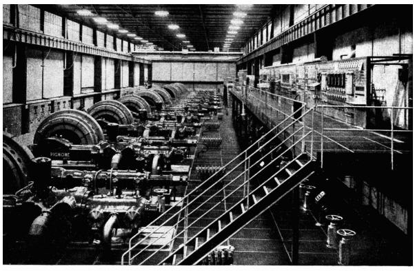
Compressor hall for ammonia synthesis plant overall capacity 34.000 HP.
