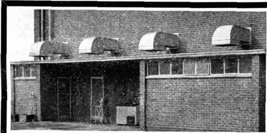
Four of the eight Colt filtered air inflow units in the No. 2 Pilot Plant at the Carrington Research Laboratories of Shell Chemical Company Ltd., nr. Manchester.
