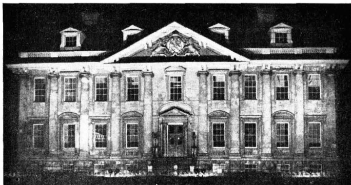
Recently installed floodlighting makes an impressive setting for Cowick Hall, Snaith, Yorks, headquarters of the Croda Organisation Ltd. (see also 'Distillates')
