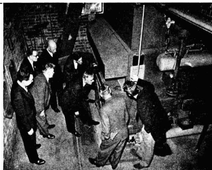
Examining a new coke-fired boiler
