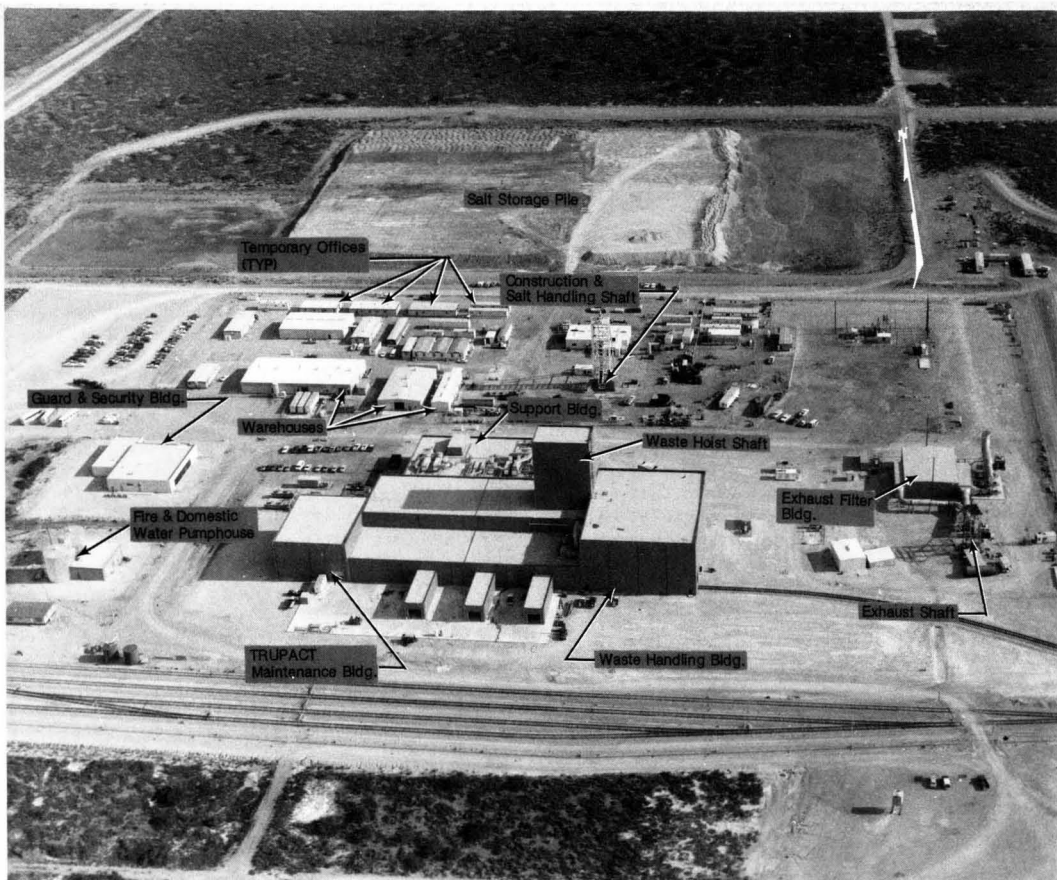
Figure 1. WIPP surface facilities.
