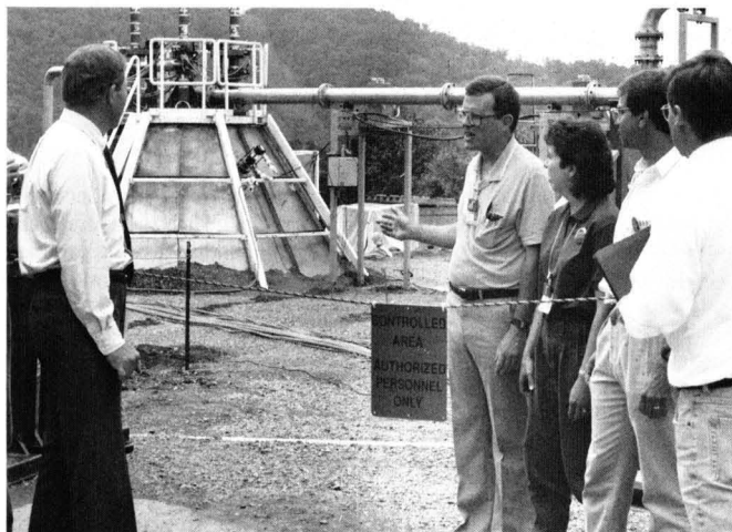
Brian Spalding, Oak Ridge National Laboratory (ORNL), Tennessee project officer for a test using electricity to melt buried waste, directs visitors' attention to the demonstration area. The test technique, known as in situ vitrification, converts old radioactive waste sites into glass by melting the contents of burial pits and trenches.
