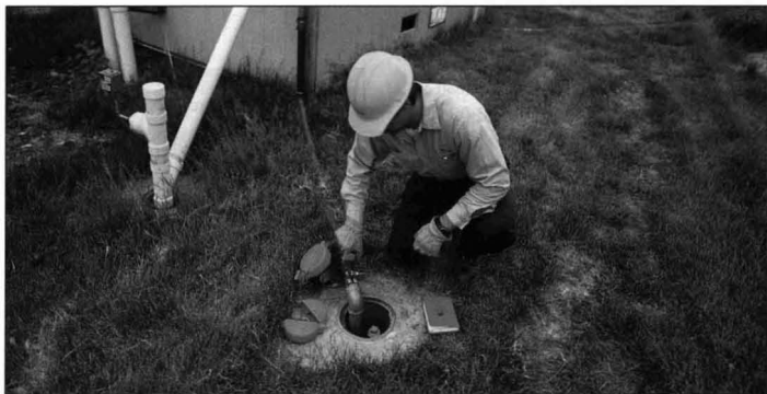
Using ozone, air sparging at one site lowered PCE levels in groundwater from 670 ppb to less than 30 ppb in 160 days.
