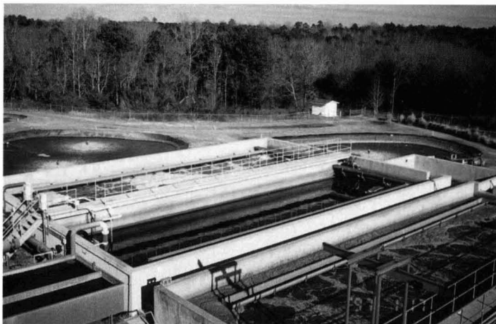
Wastewater treatment plant.
