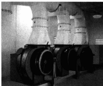
General-Purpose Fume Exhausters in a treatment-plant supply air system.
