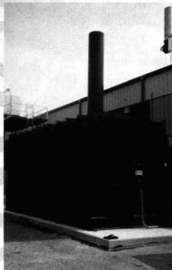
RETOX™ twin-bed RTO oxidizer designs provide up to 99 percent VOC and odor control with 95 percent primary heat recovery. The units operate fuel free at 3 percent LEL loadings. Each system is shop-assembled and skid-mounted and utilize a natural gas burner for rapid system start up. Adwest Technologies Inc. **Circle 63 on card.**
