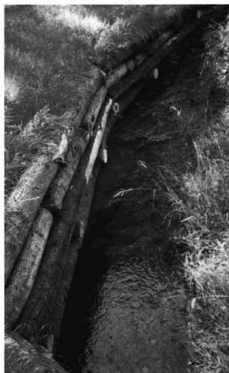
Finished cribbing with fish overhang using overhang of bottom log structure.
