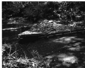
Single wing deflectors concentrate and direct flow.
