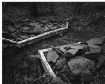
Channel constrictor installed to concentrate and direct flow through mechanically created deep pool.
