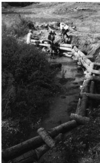
Existing exposed soils and bank required crib stabilization.
