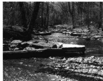
Stream meander was created by installing deflectors and constrictors in series.
