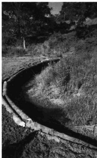
Stabilized stream bank backfilled and seeded.
