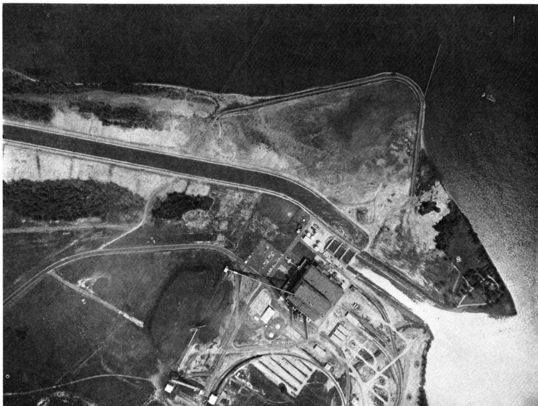
Heated effluent. At the Chalk Point, Md., generating station of the Potomac Electric and Power Co., heated water from coolant systems is pumped 2 miles upstream (canal shown at center of photo) before being discharged to the Patuxent River
