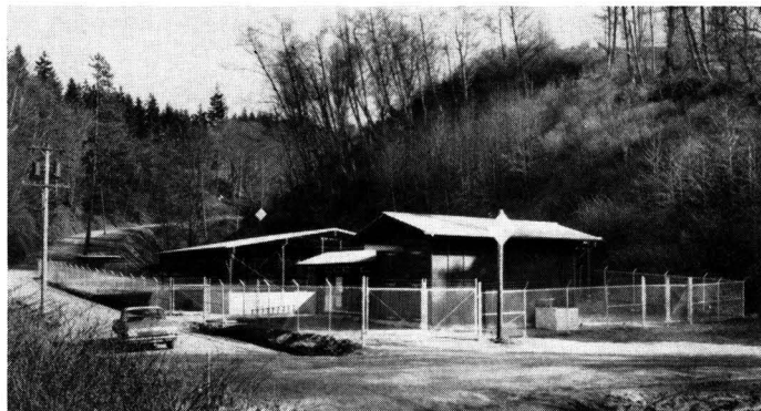
Sewage sludge. First commercial fluid bed unit for burning sewage sludge was installed at Lynnwood, Wash. Ash product from incinerator is used for landfill
