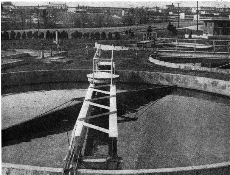
Navy. This modern installation serves the U.S. Naval Training Center at Bainbridge, Md., and includes, among other treatment equipment, primary sedimentation units, trickling filters, and prechlorination devices
