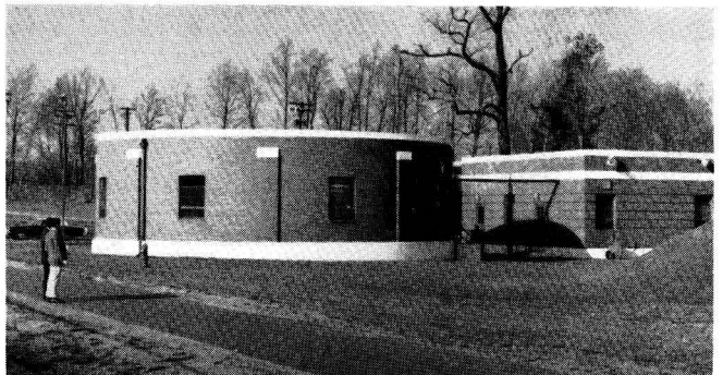
Odor. Sewage treatment operators control odor at this new Havre de Grace, Md., plant by completely enclosing treatment tanks
