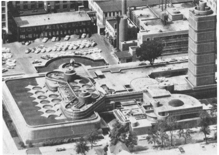
Headquarters. Catalysis is a key abatement technique at Johnson Wax's Racine (Wis.) complex, site of the company's corporate offices and research facility
