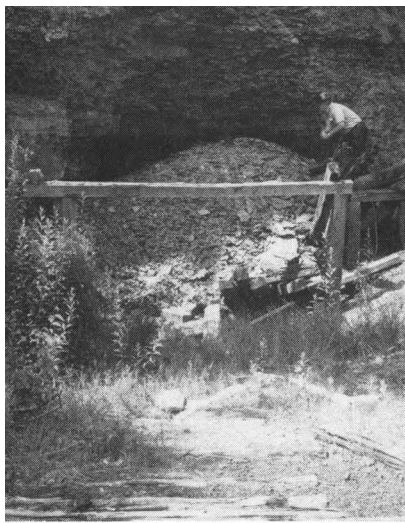
Source. Abandoned mines are more than half the problem in most states
