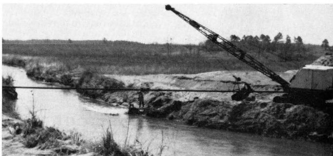
Outfall. Water effluents can be monitored under field conditions
