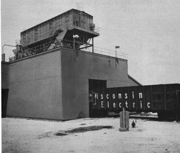
Unloading system designed by Sargent & Lundy Engineers, Chicago.
