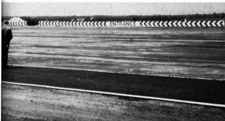
Field demonstrations. Sludge material was used for a 120-acre road bed surface at TRANSP 72, Dulles International Airport; cross section is shown of General Battery Corp.'s sludge using battery casings as aggregate
