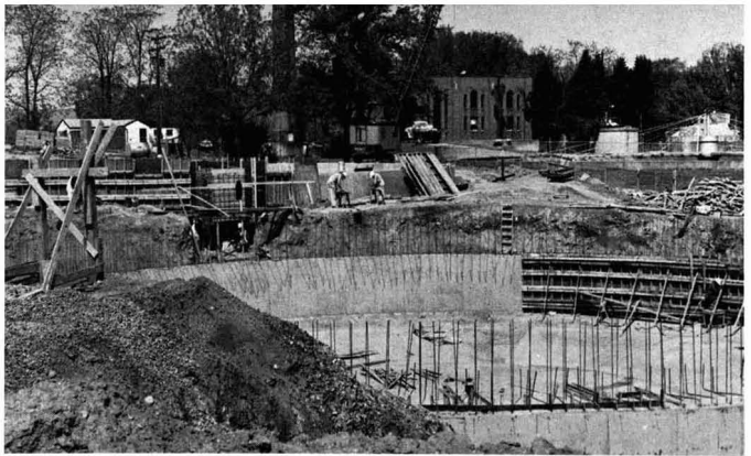
Expansion. To update sewage treatment, MES may enlarge inadequate facilities
