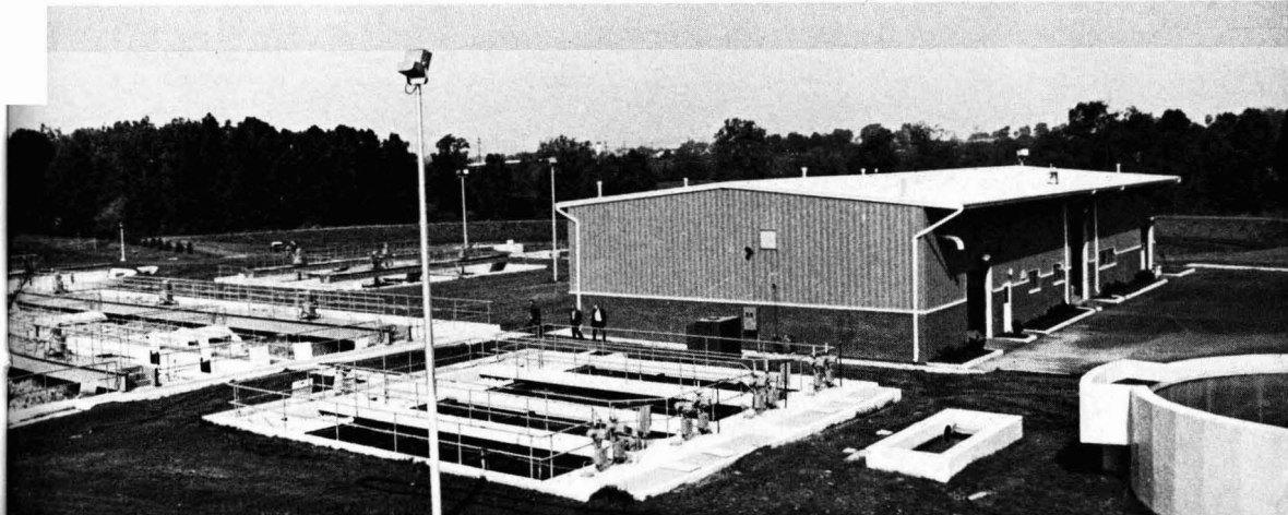
Raritan Twp. Municipleplex arranged $2.2 million worth of financing to build this treatment plant in Flemington, N.J.
