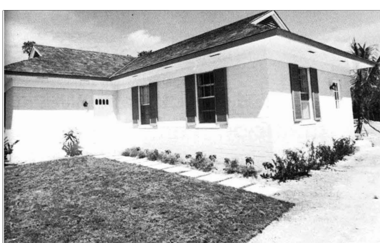
Recycling. The bricks in the house at the left were made out of ocean bottom and waste tailings. Tekology's Ryan (below) builds a model Teklokklok wall (the real thing is in the background)
