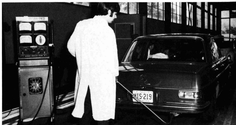
Sniffer. Technician measures tailpipe emissions at N.J. inspection station
