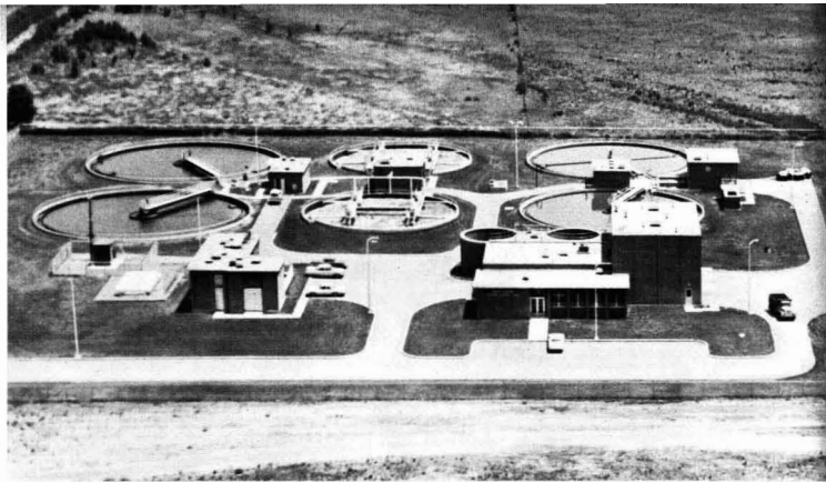
Aeration. The Grand Island, Nebraska complete mixing activated sludge plant above, like the two 0.5-mgd contact stabilization tanks at the right, can achieve about 98% BOD removal
