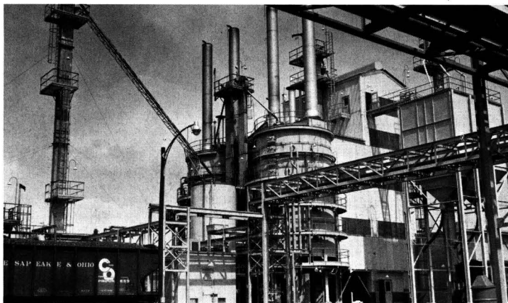
The $16-million expansion of Calgon's Big Sandy plant will be the fifth at this facility. Preliminary grading is now underway with startup scheduled for late 1975.
