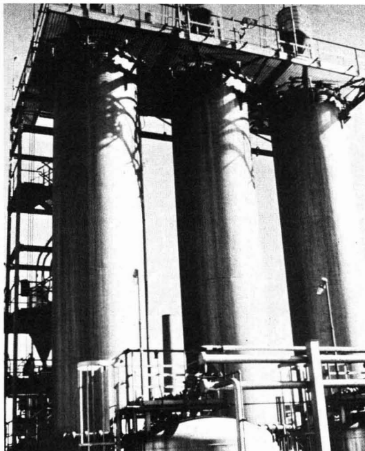
Carbon adsorption. BP Oil's refinery meets first-stage ultimate oxygen demand standards set by the Delaware River Basin Commission
