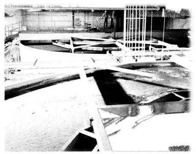
Treatment plant. Tertiary treatment removes the phosphorus from Ely's wastewater collected in these large chambers
