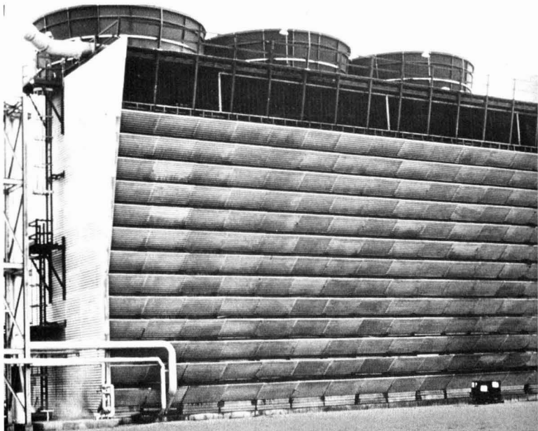
Wet/dry cooling towers. They are saving water for Consumers Power
