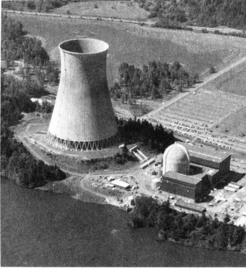
Cooling tower. Natural draft tower of the Trojan nuclear plant in Oregon tradeoffs water quality for atmospheric modification
