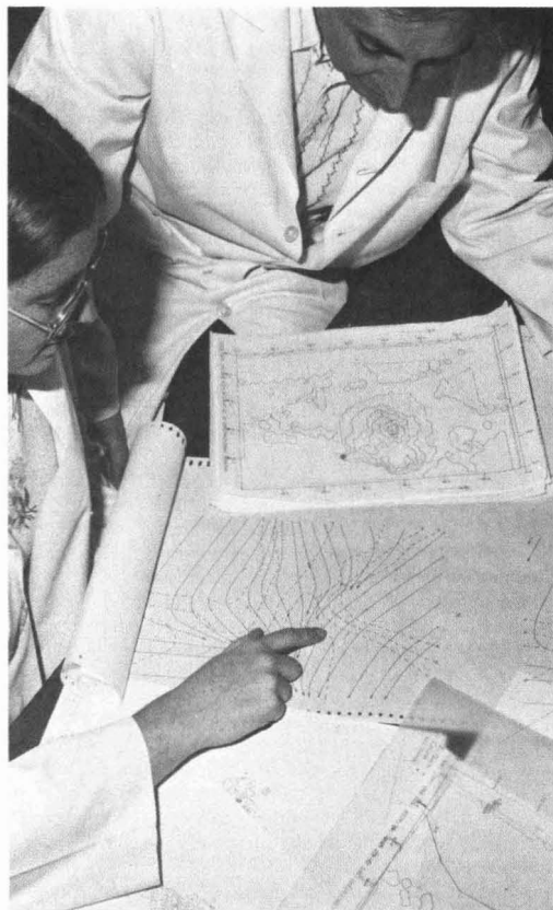
Simulation model. The model can be used to site air-monitoring stations within an airshed through the development of pollution distribution maps
