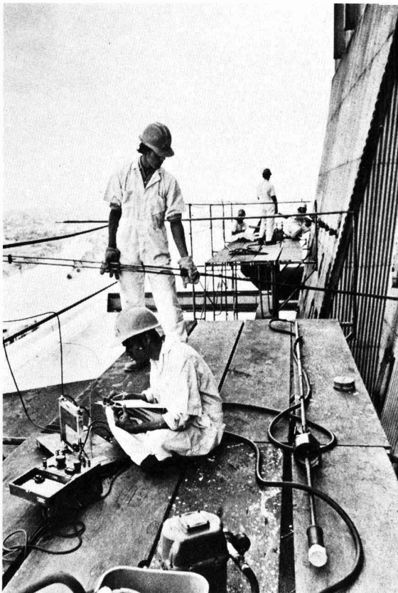
Probe. A technician takes samples from stack gases; another records the data from the instrumentation
