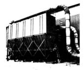
MC-1080 Aire-Vac Shaker Collector drawing off fumes from induction furnaces.
