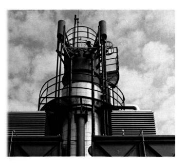
Pictured left is the 70,000 scfm PURASIV HR System recovering 2,000 lbs./hour of gravure publication printing solvents. The system is installed in the United States and went on stream in 1979.
