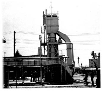
This 8,000 scfm unit at a film processing plant has been recovering about 225 lbs/hr of toluene since 1975. Foundation is  $20^{\prime} \times 20^{\prime}$ , height is about 35 $^{\prime}$ .
