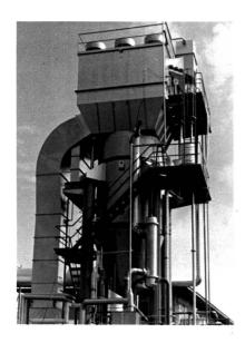
An adhesive tape manufacturing plant has employed this 29,000 scfm unit since 1976, recovering about 1,200 lbs/hr of toluene. The unit is installed on a  $30' \times 30'$  foundation and is about 50' high.
