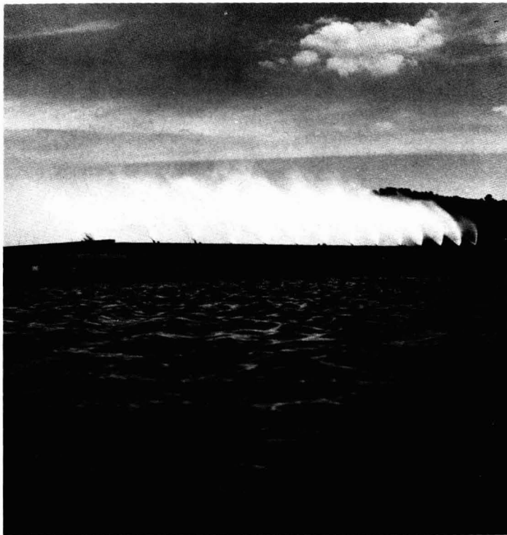
Drinking water being double aerated to remove volatile contaminants
