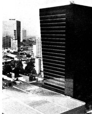
Solar collector array
