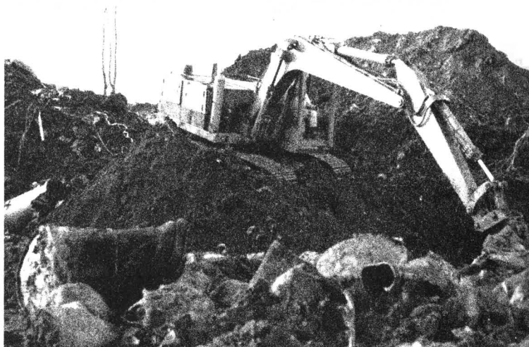
Hazardous wastes are removed from a Minnesota site
