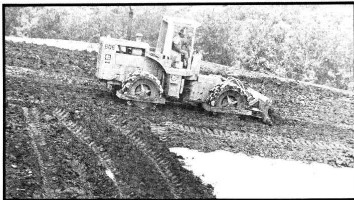
A hazardous waste site is sealed with clay and textiles
