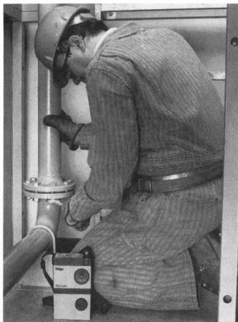
Hazardous-gas alarm system
