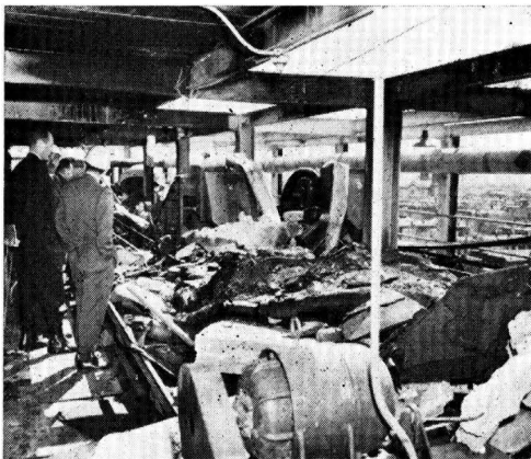
Fig. 4. Remains of the conveyor belts above the production bins
