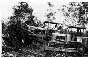
A Fowler Challenger 33 and a Track-Marshall both fitted with Marshall hydraulic angledozers working together to clear bush during extensions to sugar plantations on the Leonora estate of the Demerara Company, Guyana.
