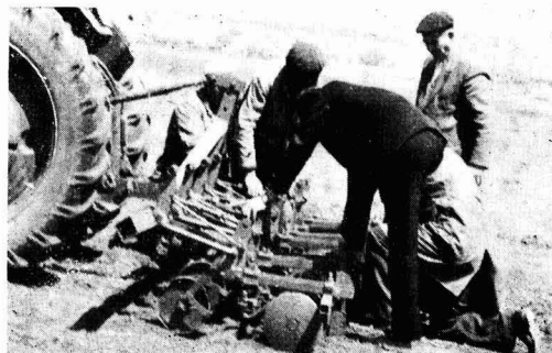
Fig. 3. Mounting of protective discs and hoe blades
