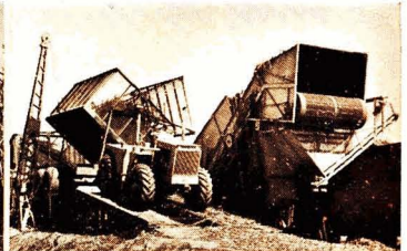
ATLAS DRY-CLEANER TRANSLOADER , removes up to 85% of fine trash and dirt (up to 65% of all extraneous matter) to give top economies in freight and at the mill. Rigged for 24 hour operation.
